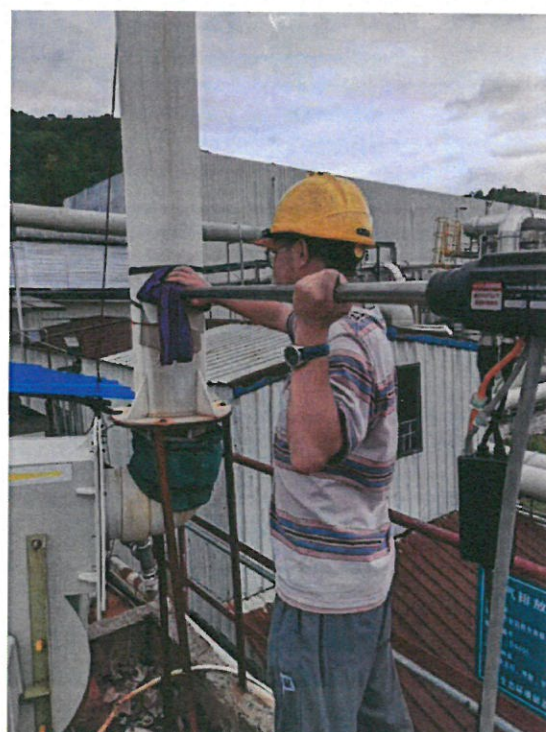
污水处理废气排气筒出口(FQPK-0005)G5
