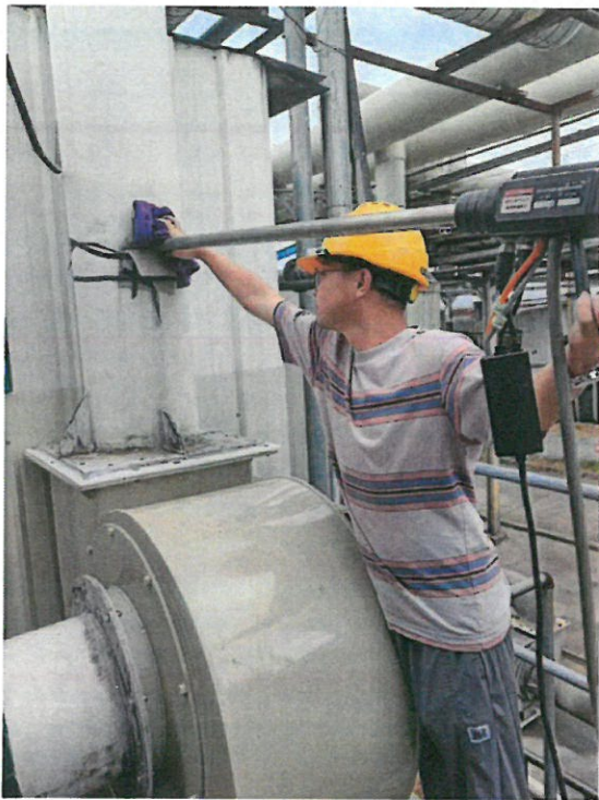
污水处理废气排气筒出口(FQPK-0006)G6
