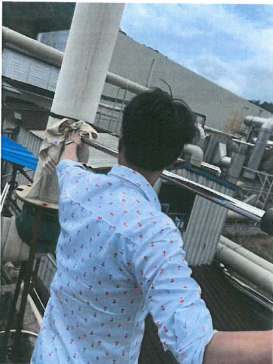
污水处理废气排气筒出口(FQPK-0005)G5
