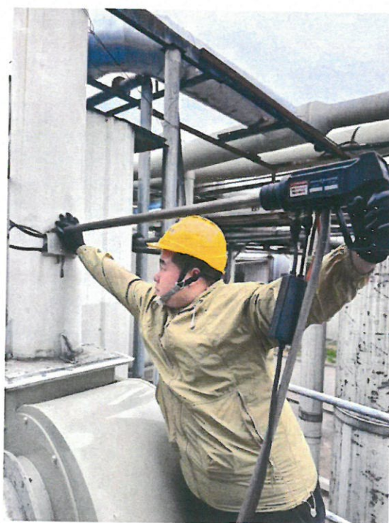
污水处理废气排气筒出口(FQPK-0006)G6
