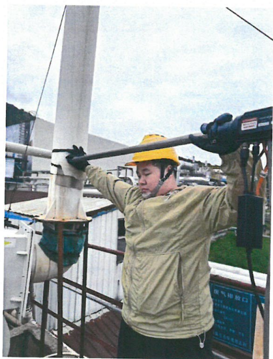
污水处理废气排气筒出口(FQPK-0005)G5
